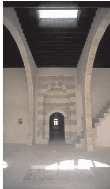
Skylight that Mirza Mihdi fell through
